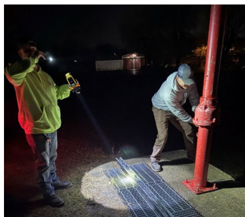
Closing a floodgate in Middletown
