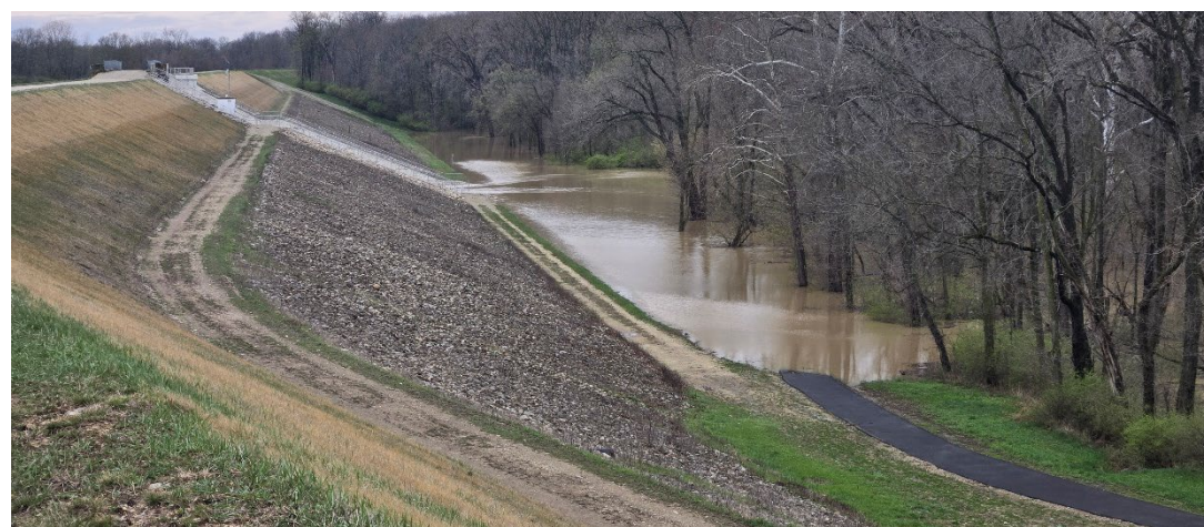
Lockington Dam Storage Basin
