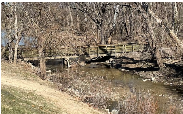
Old Bridge. Notice the middle pier and low clearance over the creek.
