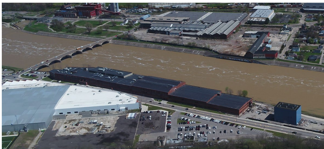
Hamilton, Black Street Bridge
