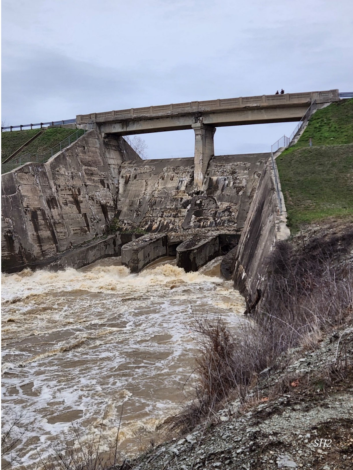
Huffman Dam, downstream
