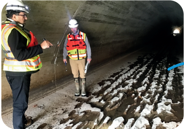
Engineers inspect the severely eroding floor of the tunnel that runs inside the Germantown Dam.
