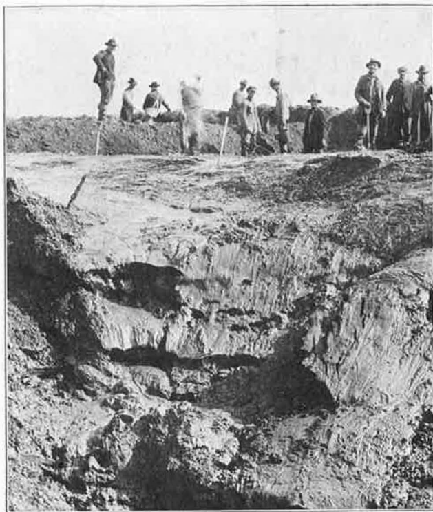
FIG. 345.—CORE EXPOSED AT ENGLEWOOD, OCTOBER 26, 1921.
