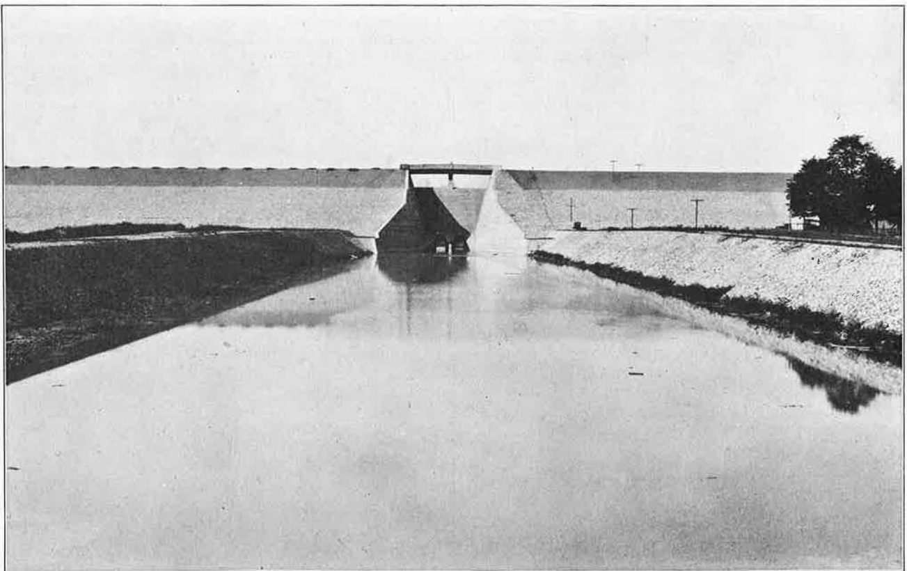
FIG. 329.—LOCKINGTON DAM COMPLETED, SEPTEMBER 28, 1921.
