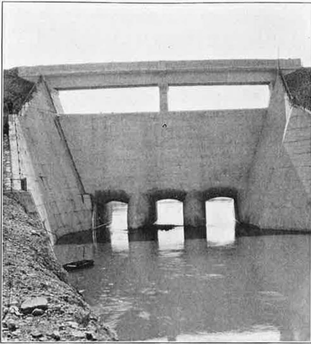
FIG. 355. HUFFMAN SPILLWAY AND BRIDGE, MARCH 22, 1922.
