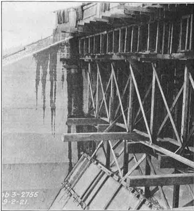
FIG. 359. BRIDGE FORMS AT LOCKINGTON, SEPTEMBER 2, 1921.
