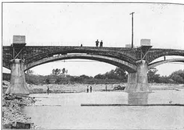
FIG. 391—ADAMS STREET BRIDGE, AUGUST 21, '22.
