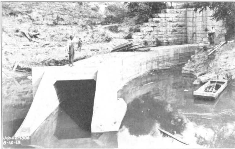
FIG. 47—THE MCKINLEY PARK SEWER EXTENSION, AUGUST 12, 1919.
