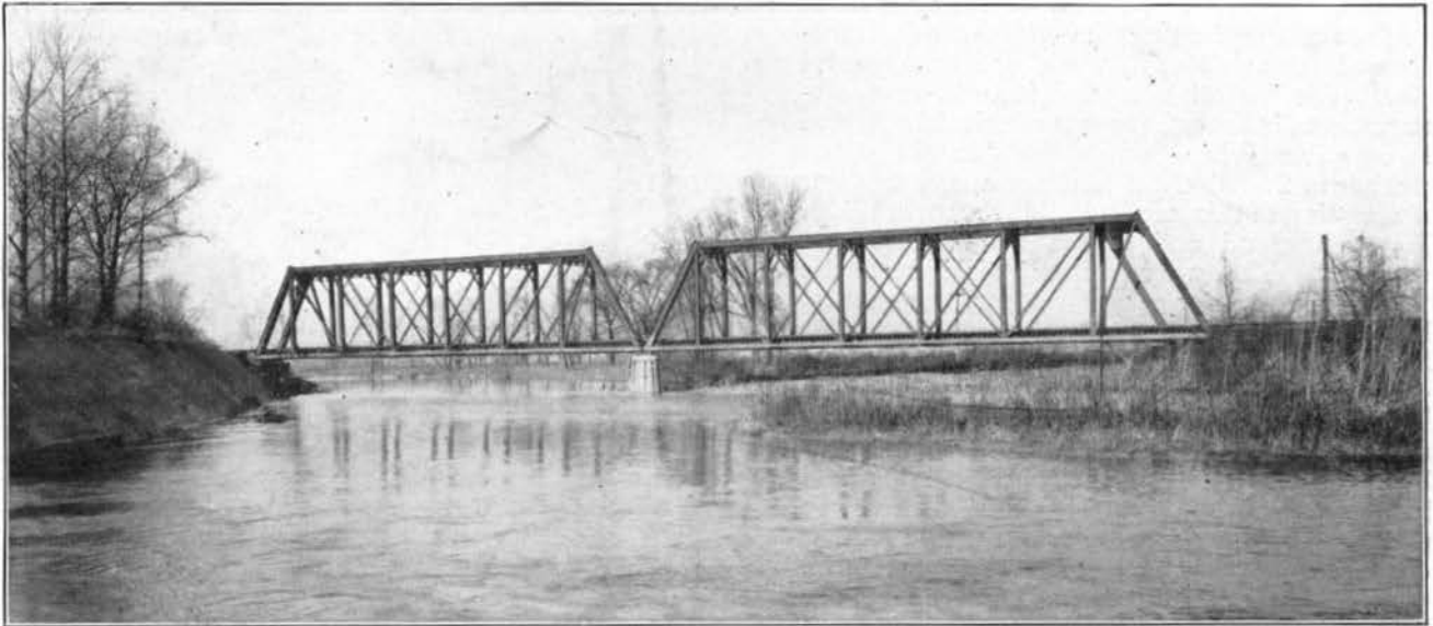
FIG. 122—ERIE RAILWAY BRIDGE OVER MAD RIVER
