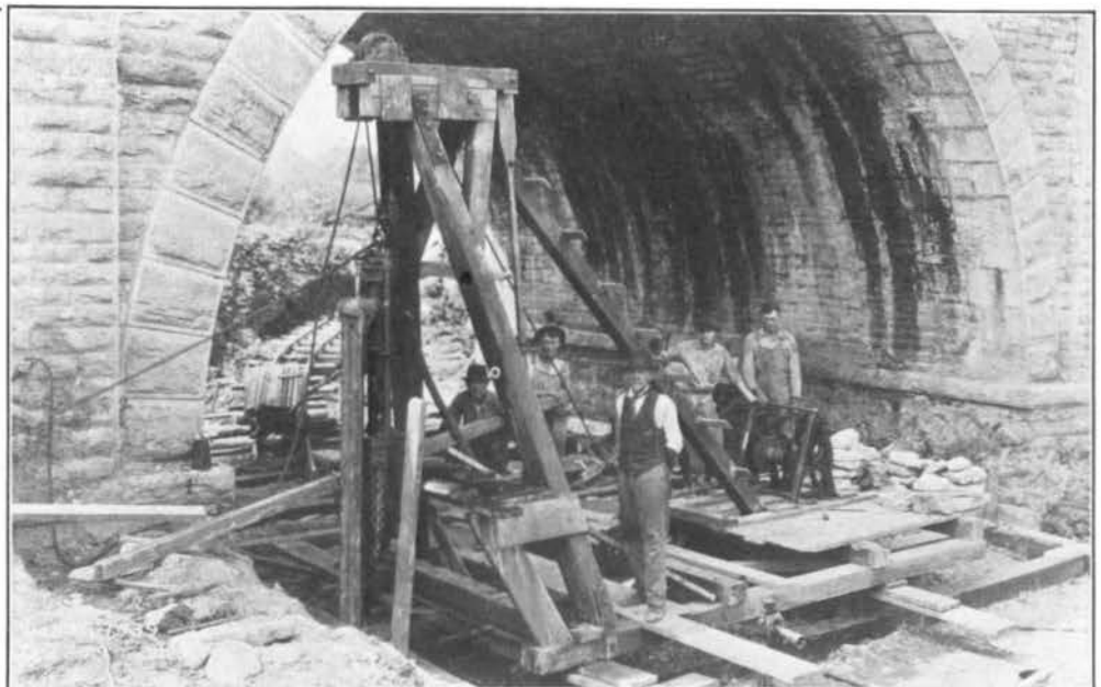
FIG. 154—DRIVING SHEET PILING FOR TAILRACE CONDUIT FOUNDATIONS, AUGUST 22, 1919
