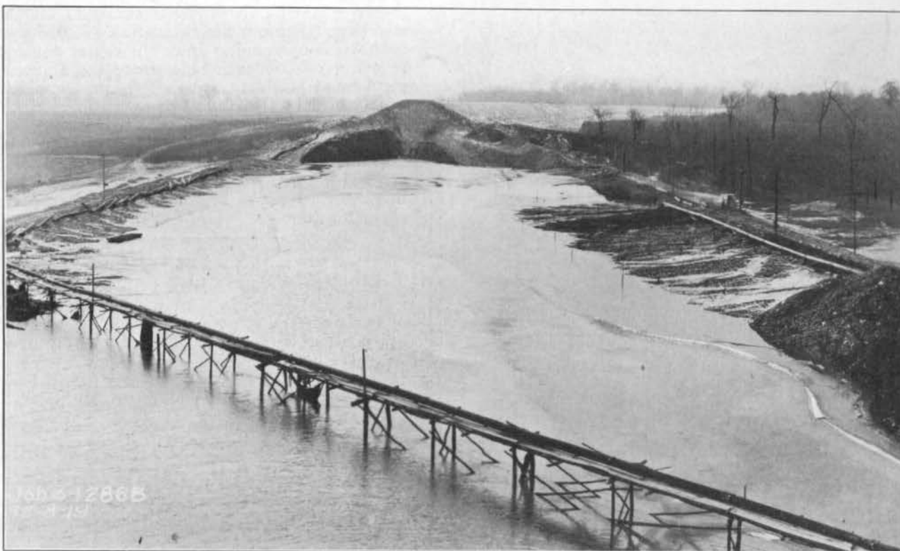
FIG. 81—LOCKINGTON DAM EMBANKMENT, DEC. 8, 1919.
