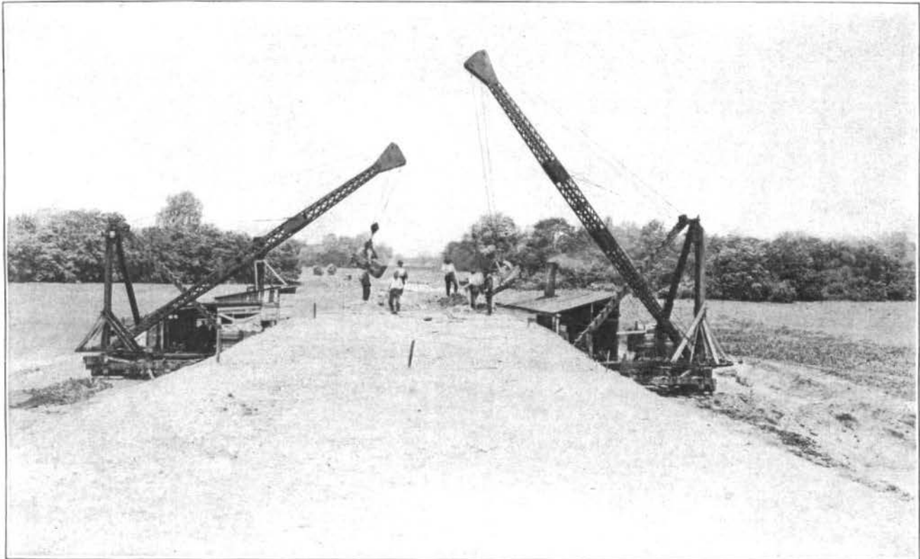
FIG. 65—TEAM OF DERRICK DRAGLINES BUILDING OHIO ELECTRIC RAILWAY EMBANKMENT
