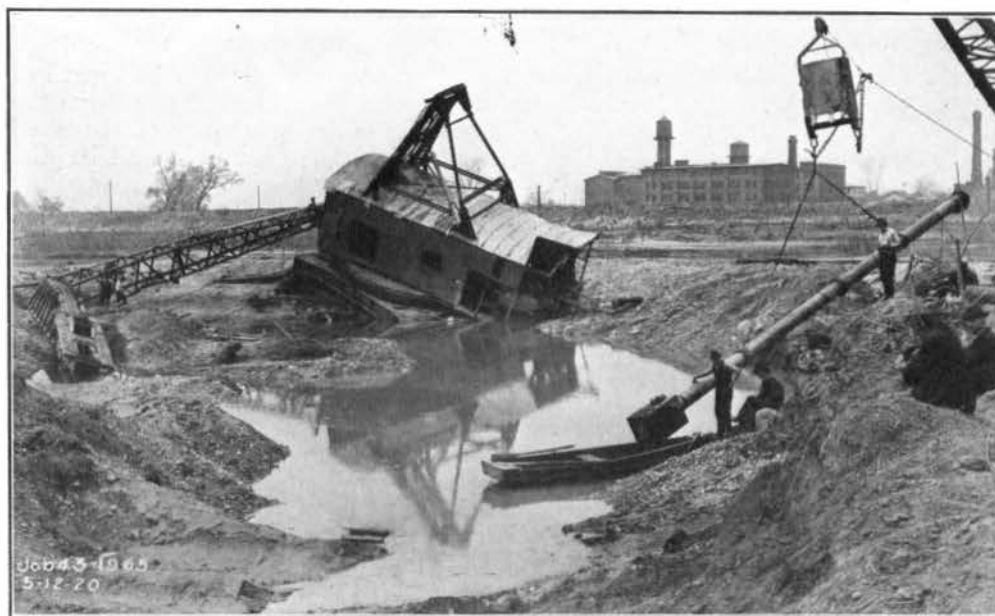
FIG. 146—WRECKED DAYTON DRAGLINE EXCAVATOR, MAY 12, 1920.
