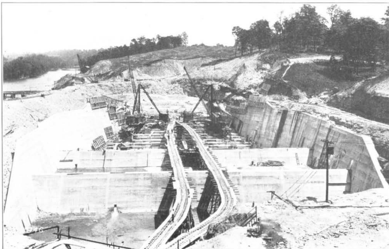
FIG. 151—DOWNSTREAM END, OUTLET STRUCTURE, TAYLORSVILLE DAM, JUNE 11, 1920.
