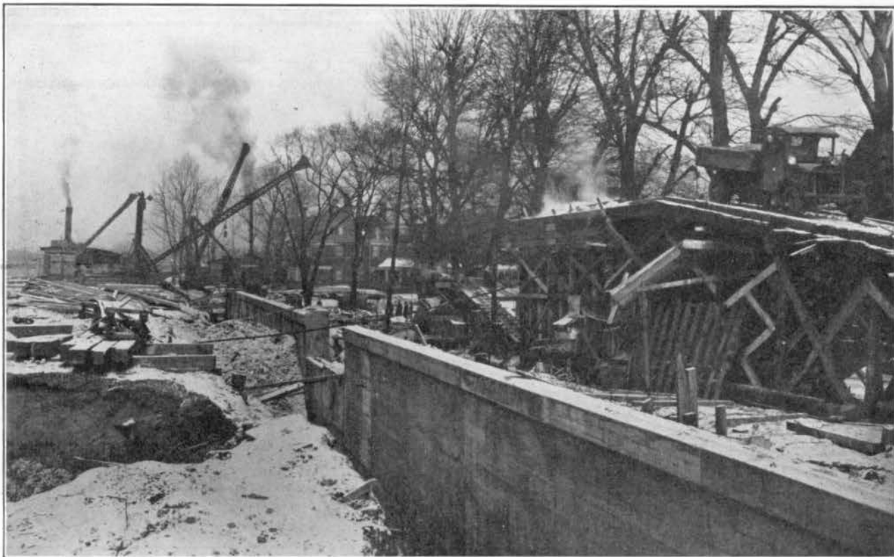
FIG. 100—CONCRETING PLANT, ROBERT BOULEVARD WALL, DAYTON, FEB. 19, 1920.
