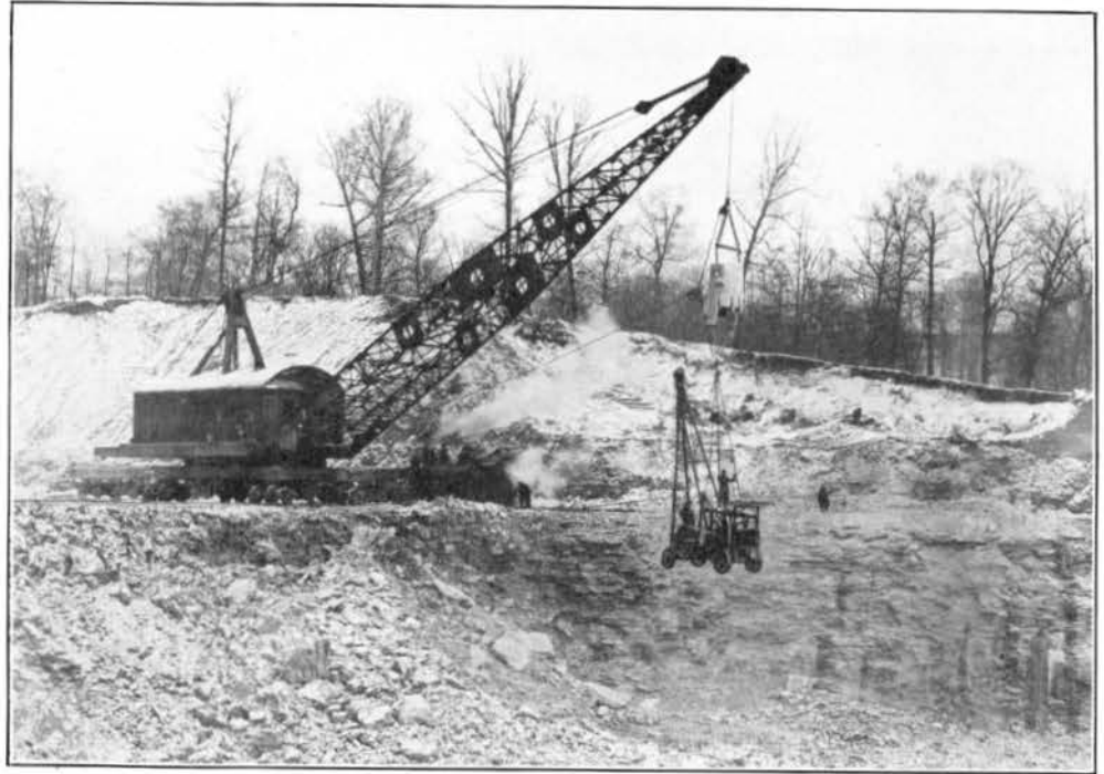
FIG. 77—LIDGERWOOD DRAGLINE LIFTING WAGON DRILL, TAYLORSVILLE DAM.
