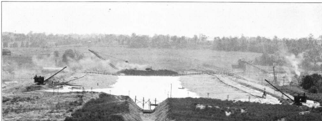
FIG. 90—CORE POOL, BEACHES, PIPE LINES, AND LEVEES, ENGLEWOOD DAM, AUGUST 26, 1919
