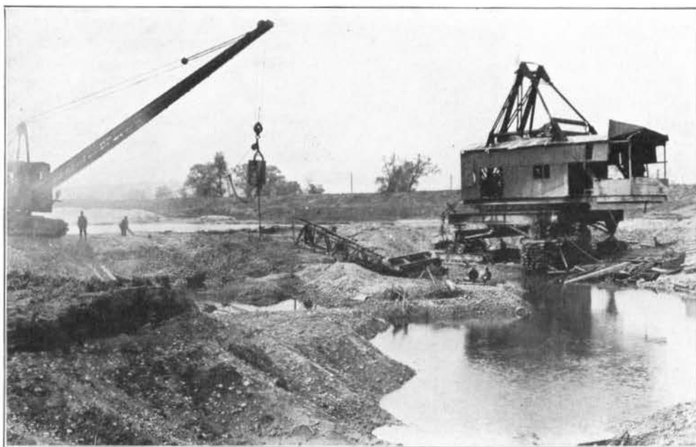
FIG. 147—WRECKED DAYTON DRAGLINE EXCAVATOR, MAY 27, 1920.
