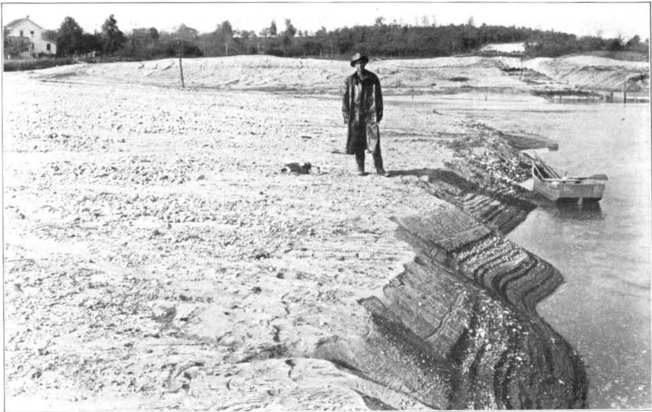
FIG. 87—BEACH AND SLOPE AT EDGE OF POOL, ENGLEWOOD DAM, MAY 26, 1919
