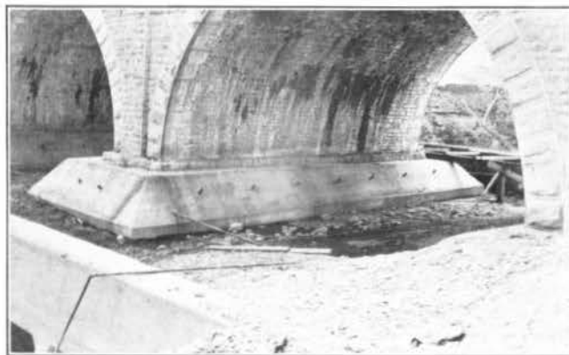
FIG. 158—CONCRETE REINFORCING BRIDGE PIER, JUNE 23, 1920
