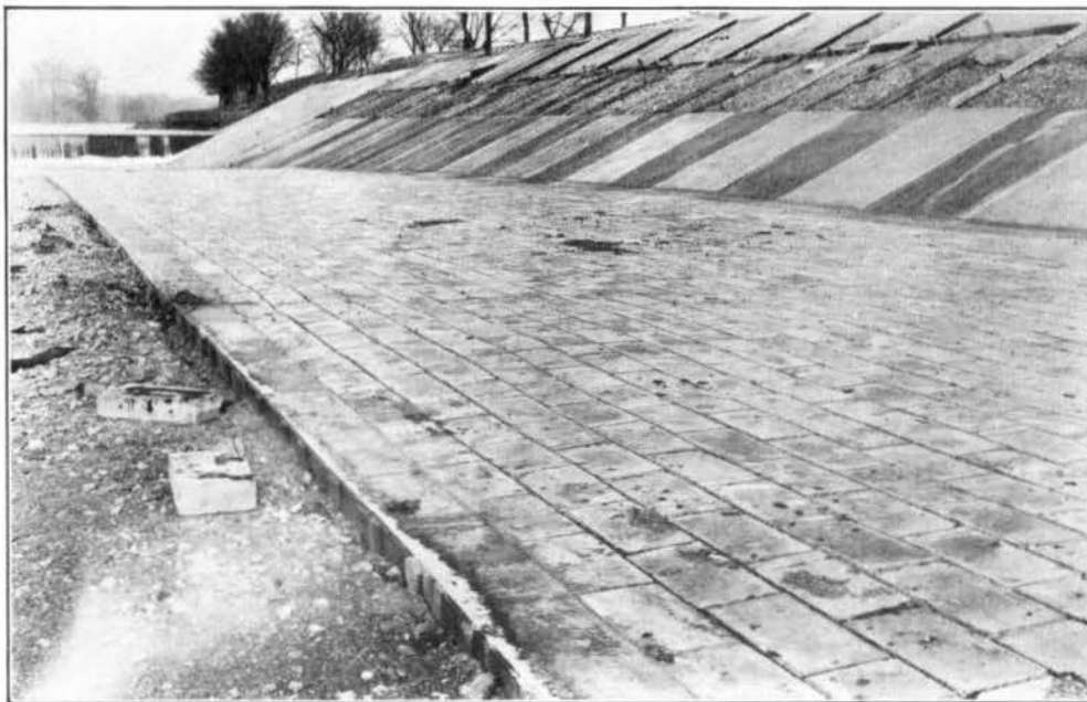
FIG. 76—CONCRETE REVETMENT, MIAMI RIVER AT DAYTON, DEC. 29, 1919.
