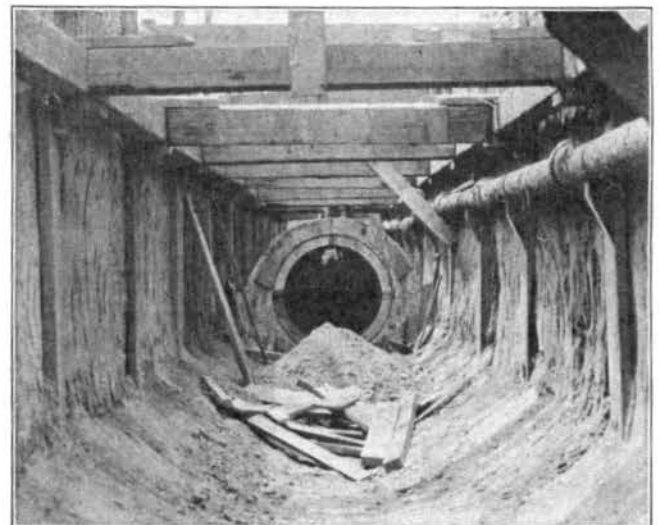
FIG. 59—WOOD ST. SEWER TRENCH, HAMILTON
