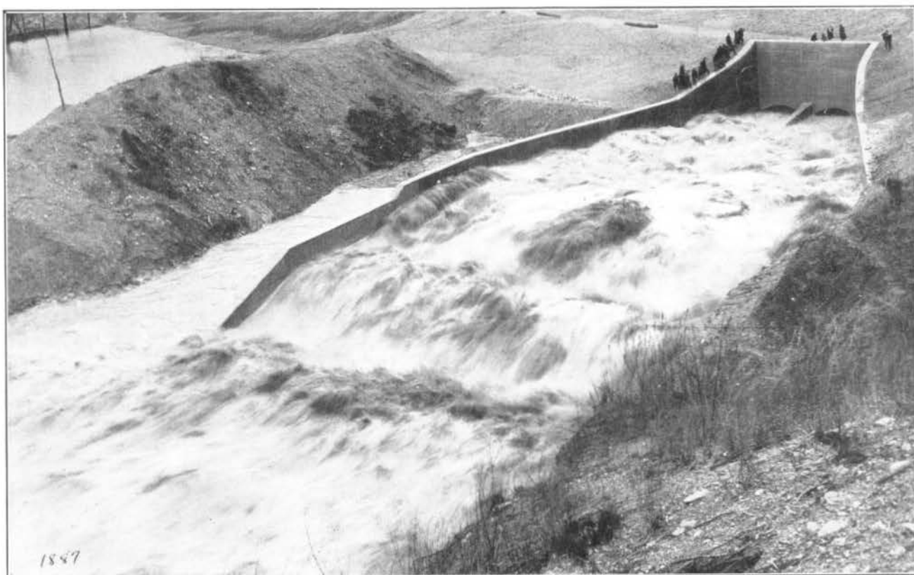
FIG. 123—HYDRAULIC JUMP AT GERMANTOWN DAM OUTLET, APRIL 20, 1920.
