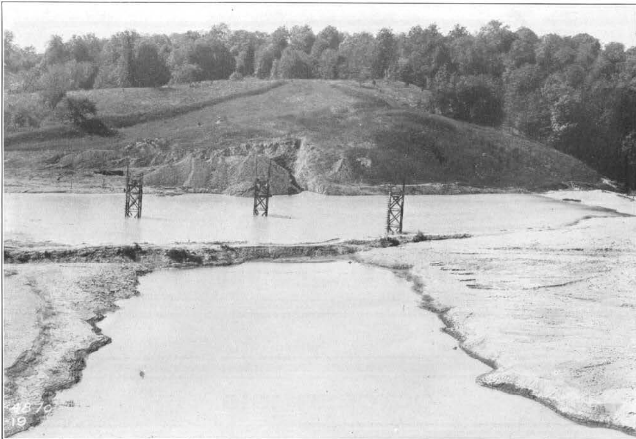
FIG. 29—HYDRAULIC FILL POOL AT GERMANTOWN DAM, SHOWING PRESSURE CELL TOWERS
