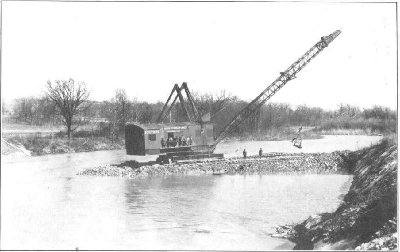
FIG. 149—DRAGLINE EXCAVATOR CROSSING STILLWATER RIVER AT ENGLEWOOD. MARCH 3, 1920.
