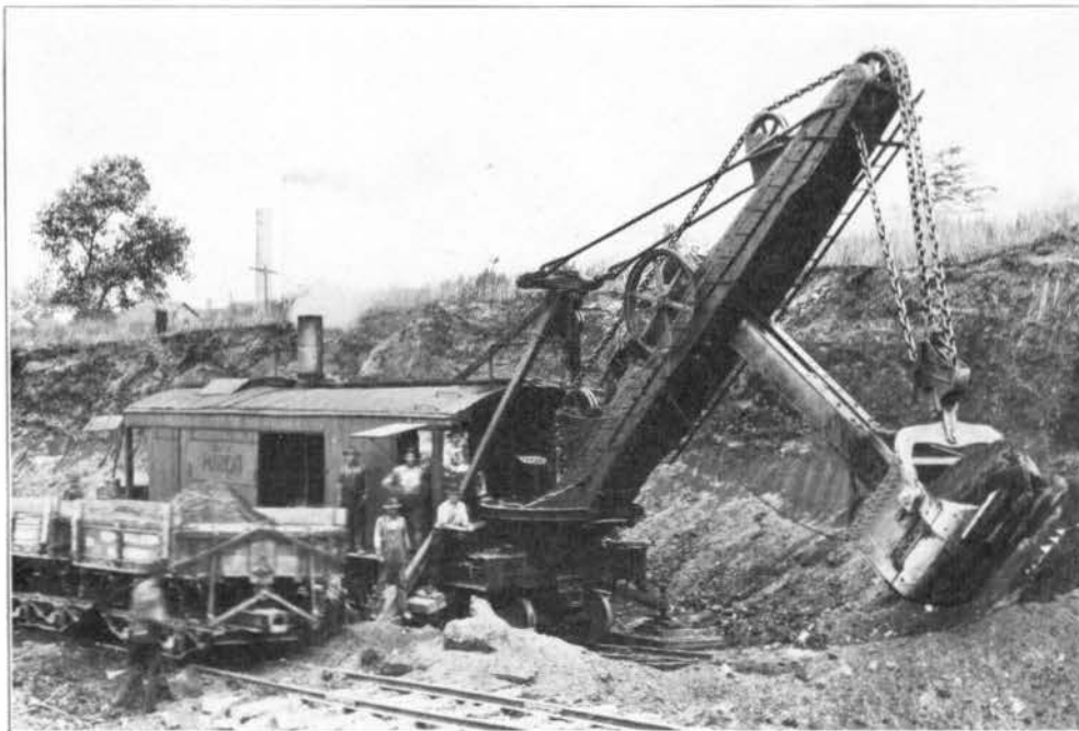
FIG. 79—STEAM SHOVEL AT HAMILTON, SEPT. 11, 1919.
