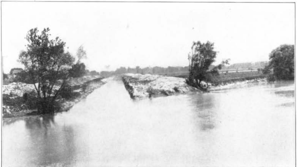
FIG. 162—THE NEW CUTOFF CHANNEL BELOW TROY
