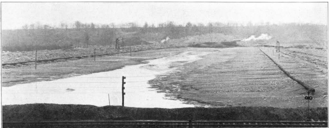
FIG. 96—CORE POOL AND BEACHES, TAYLORSVILLE DAM, DECEMBER 1, 1919.
