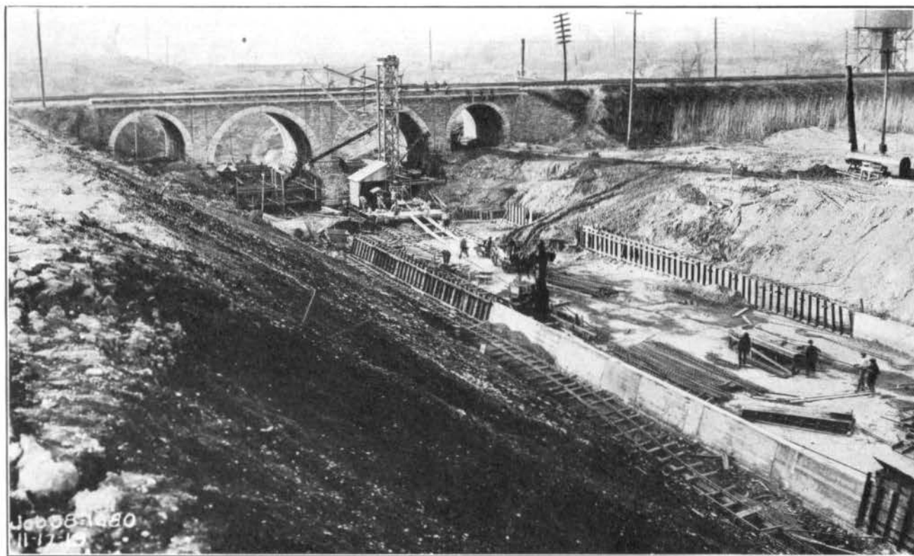
FIG. 73—BUILDING TAILRACE UNDER B. & O. R. R. BRIDGE, HAMILTON, NOV. 17, 1919.
