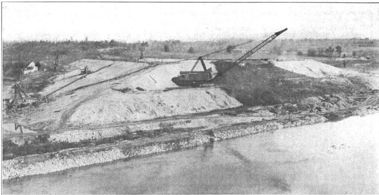
FIG. 55—BUILDING FIRST SECTION, ENGLEWOOD DAM, NOV. 11, 1919
