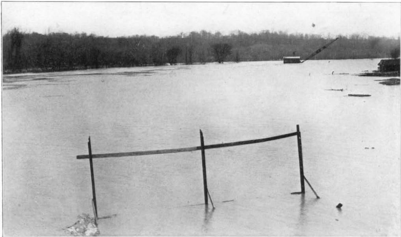
FIG. 126—DRAGLINE EXCAVATOR "AFLOAT" ON THE FLOOD, APRIL 20, 1920.
