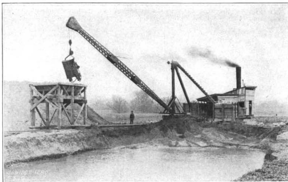
FIG. 64—DERRICK DRAGLINES LOADING CONCRETE GRAVEL, MAY 5, 1919
