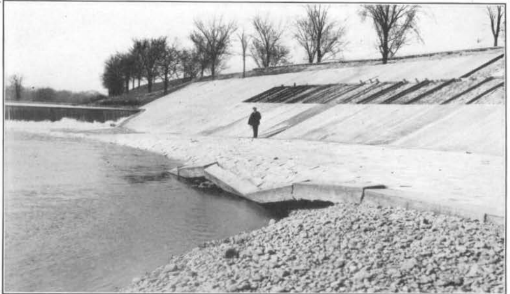
FIG. 144—THE FLEXIBLE REVETMENT IN ACTION. MARCH 25, 1920.
