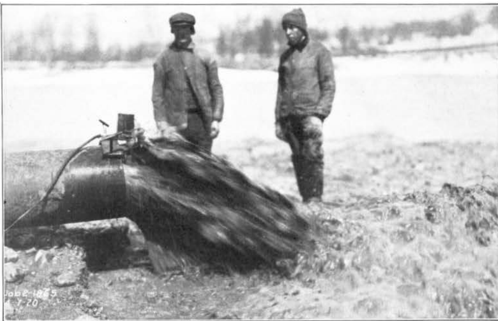
FIG. 140—DISCHARGE END OF DREDGE PIPE LINE AT ENGLEWOOD DAM, APRIL 7, 1920.
