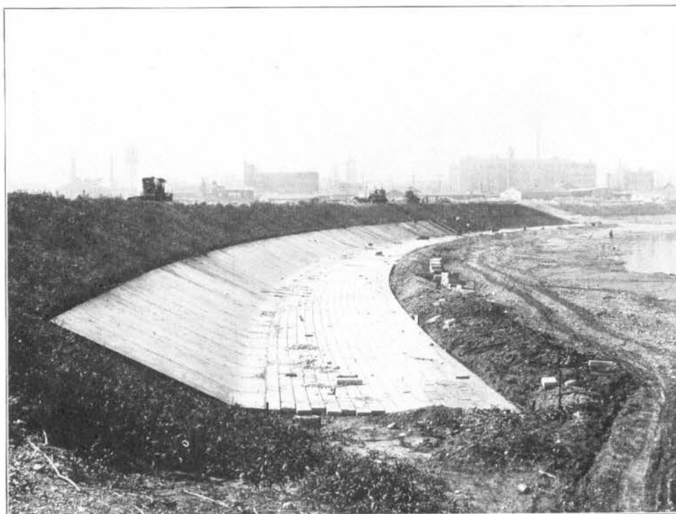
FIG. 143—FINISHED SECTION OF CONCRETE REVETMENT, MAY 26, 1920.
