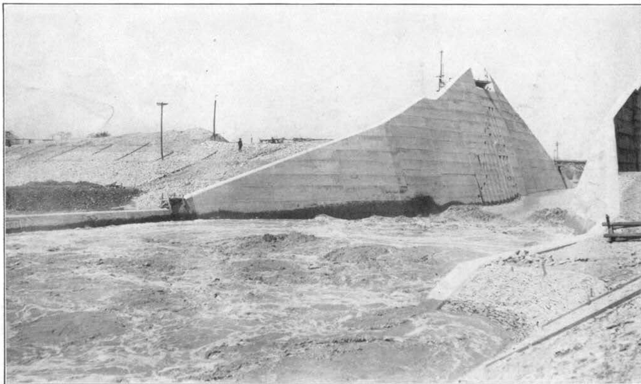
FIG. 135—HYDRAULIC JUMP AT LOCKINGTON DAM, APRIL 20, 1920, LOOKING UPSTREAM
