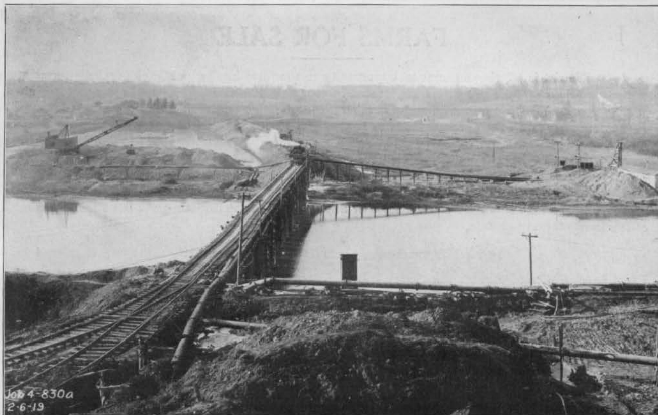
FIG. 97—PIPE LAYOUT AND CROSS DAM, TAYLORSVILLE DAM, FEBRUARY 6, 1919
