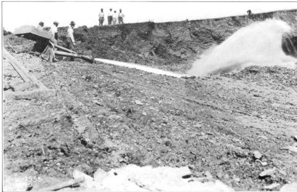
FIG. 35—HYDRAULICKING DOWN HILLSIDE AT GERMANTOWN
