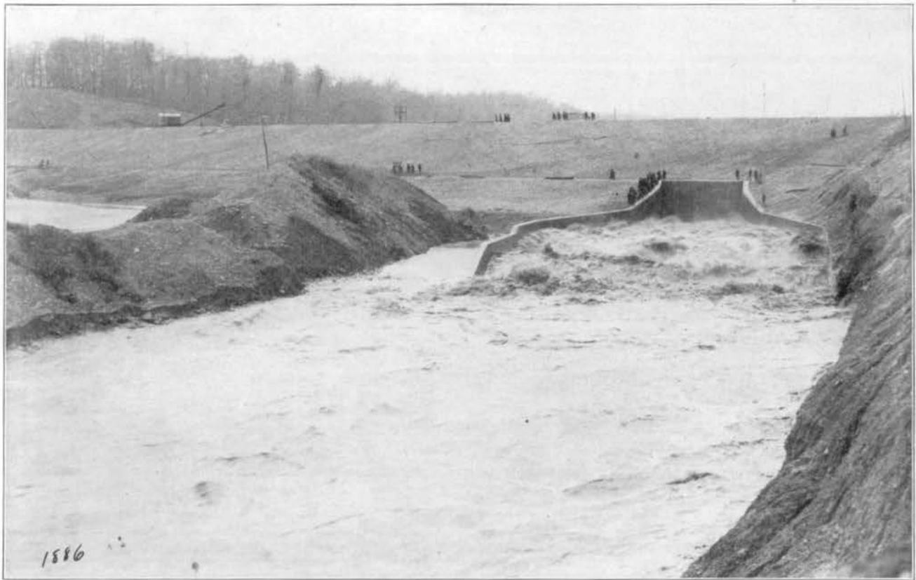
FIG. 124—HYDRAULIC JUMP AT GERMANTOWN DAM OUTLET, APRIL 20, 1920.
