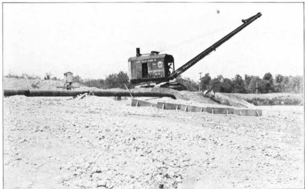
FIG. 92—BUILDING LEVEE AT ENGLEWOOD DAM, JULY 28, 1919
