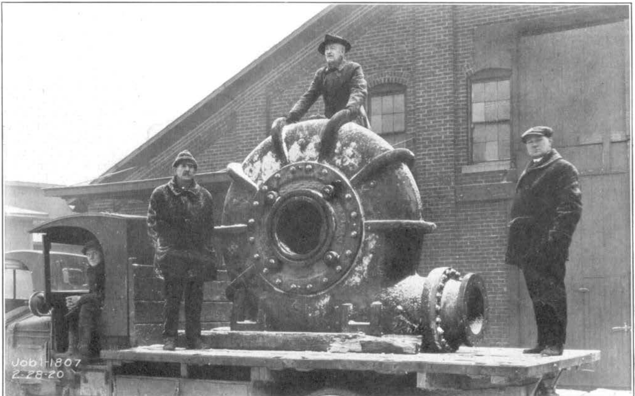
FIG. 150—HEAVY WHITE IRON CENTRIFUGAL PUMP SHELL. FEBRUARY 28, 1920.
